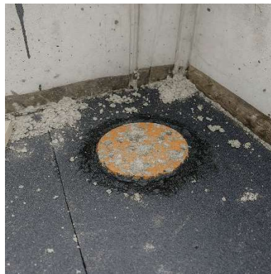
Figure 2 Sealing with waterproofing compound for a pipe socket flush with the floor slab
