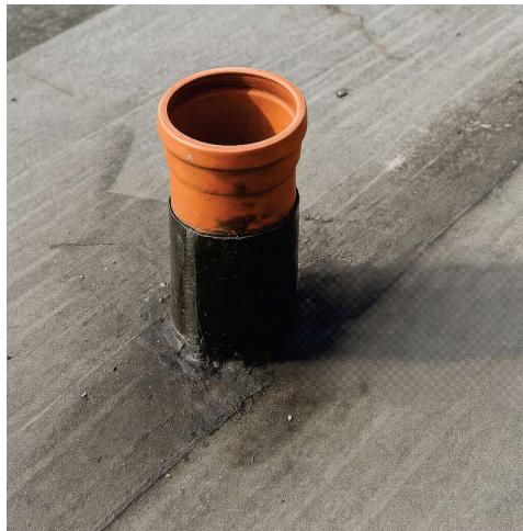
Figure 3 Raising of bitumen on the pipe feedthrough
